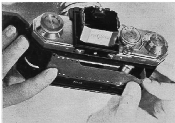
To open the camera back, pull the latch (1) outwards. Pull out rewind knob (3). Place the fresh film cartridge into the empty film chamber (4) with the film leader in the direction of the take-up spool (7). Push the rewind knob down, thus engaging the film cartridge. Pull the film from the cartridge and place the tongue into the slit of the take-up spool (7). Then turn the take-up spool by hand without using the lever, wrapping some film around the spool.
