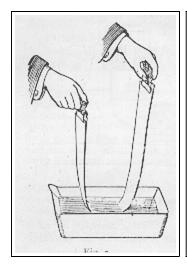
**TO DEVELOP IN THE STRIP-** In the red light unroll the spool and separate the sensitive film from the paper. Attach an "Ensign "Clip to each end of the film and holding each clip as in Fig. 7 pass the film, dull side up, through the various solutions. The clips may be left on the films until dry.
