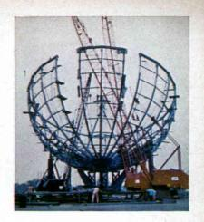
less steel; and the 3-ton stainless steel orbital rings are held in place with an almost invisible spider web of super-strong stainless steel wires, much as a bicycle wheel is anchored to the hub.
