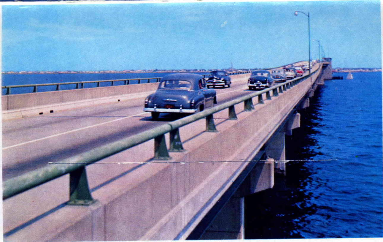
MEMORIAL BRIDGE ACROSS BARNEGAT BAY
