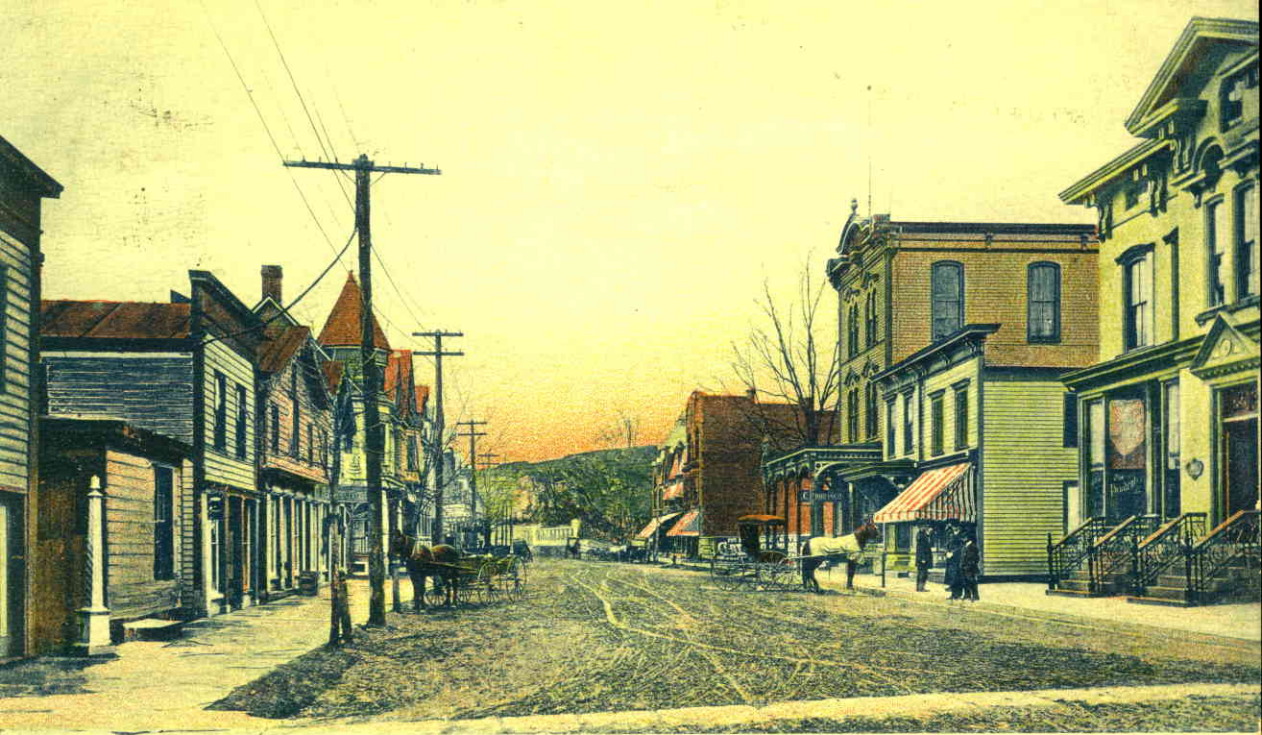
Main St. looking West from corner Leigh St., Clinton, N. J.
