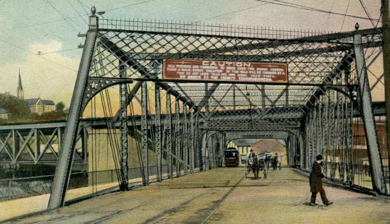
Easton, Pa. Road Bridge.
