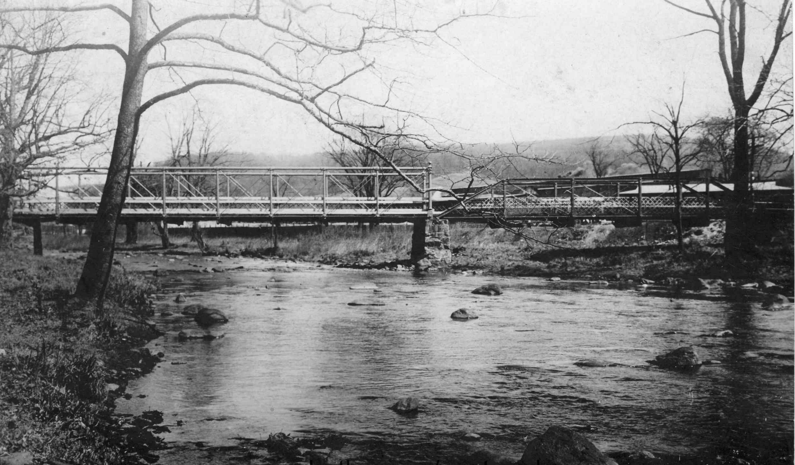
4542 Foundry Bridge. High Bridge N. J.
